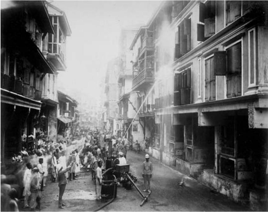
**Figure 1:** Flushing engine cleansing infected houses.
